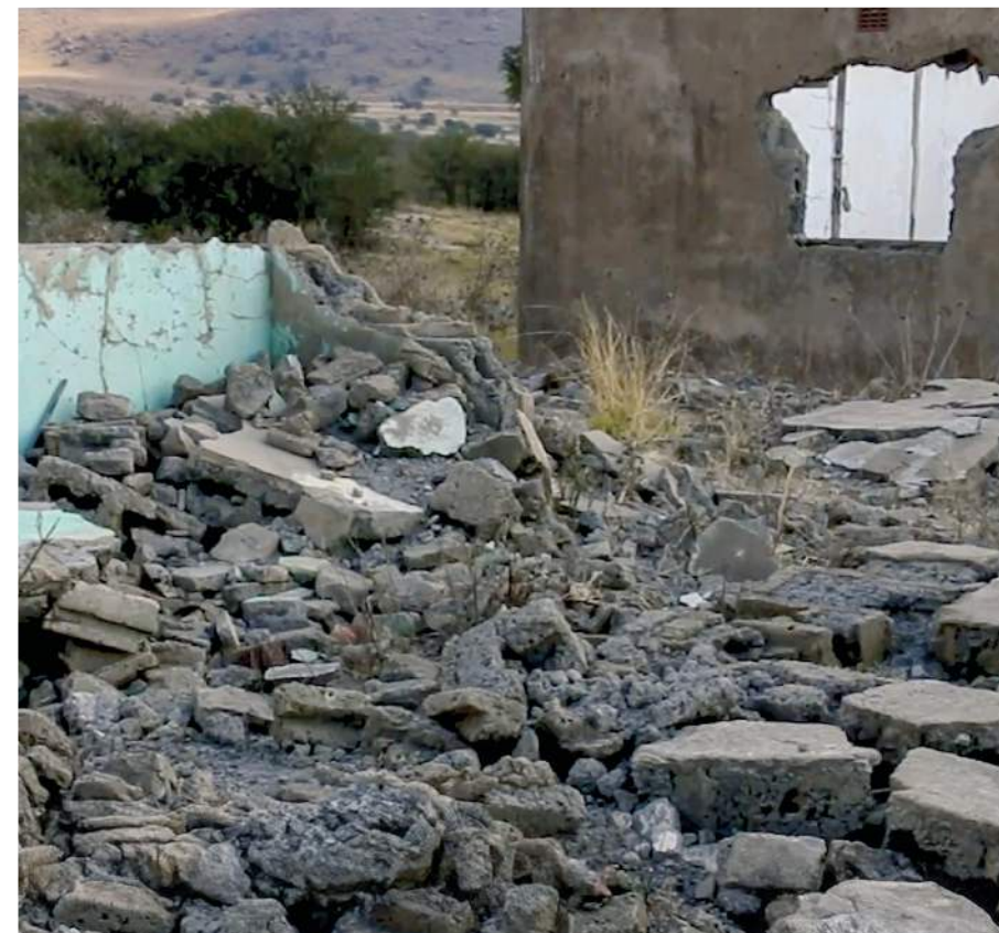
Damage to homes in New Castle as a result of coal mining activities. Screenshot from New Castle Video , produced by Corruption Watch.
